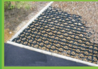
Ground reinforcement block
